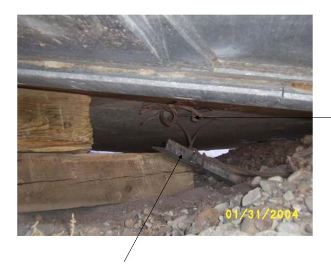
Eye plate where the cable was looped through and attached to anchor.
