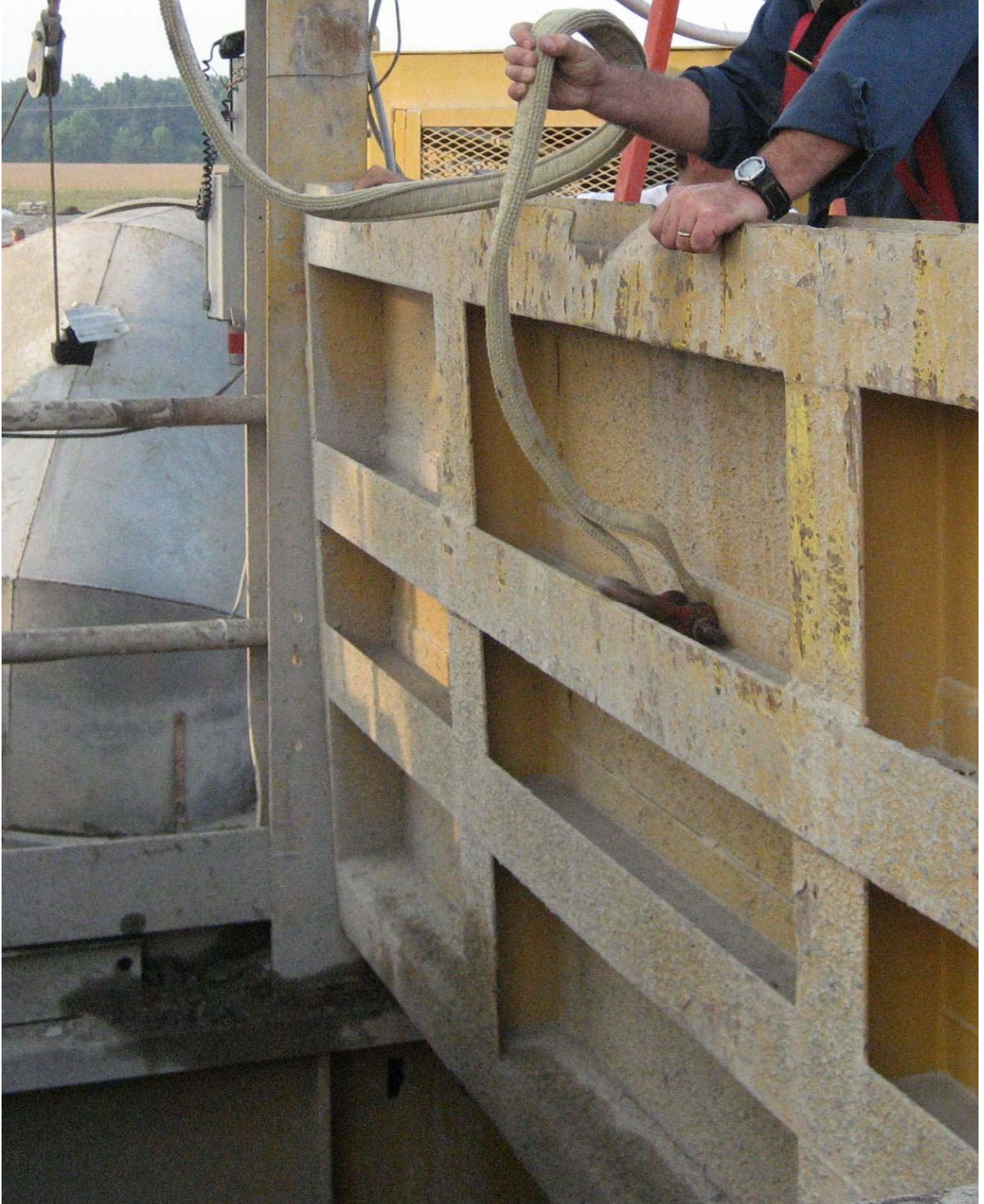
EXHIBIT 3 PHOTO OF NYLON SLING AND SHACKLE IN COLLAR DOOR
