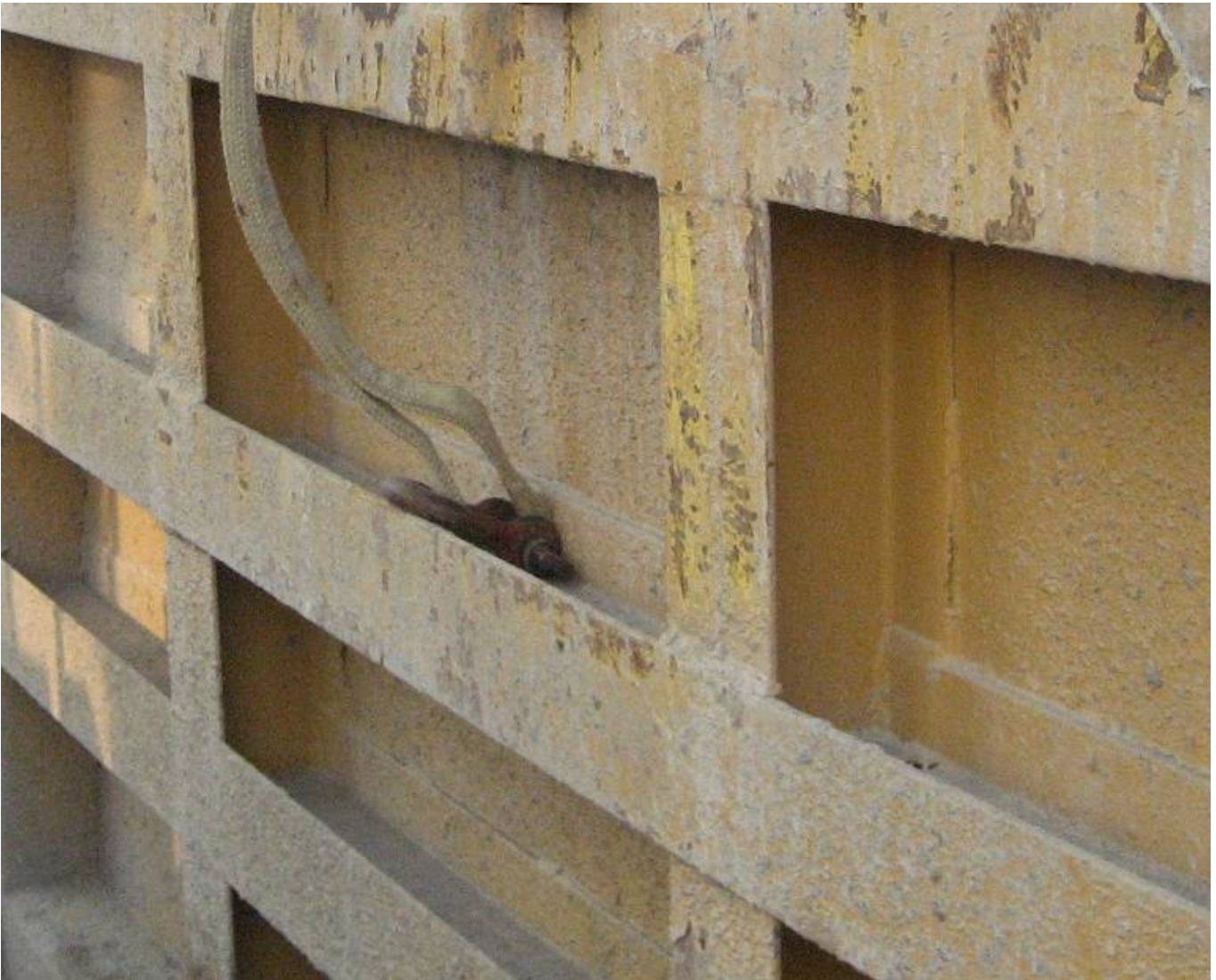
EXHIBIT 6 PHOTO OF POSITION 3 OF SHACKLE IN COLLAR DOOR
