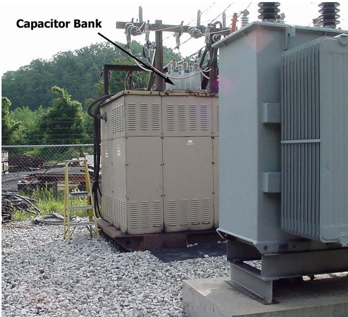
Mountain Spring Coal Company #1 Mine, I.D. No.36-08725 Beaver County, Pennsylvania Enclosed Unit with Capacitor Bank
