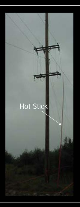
The foreman watched from the ground as the lineman, who was not a certified electrician, installed the splice within close proximity to the line side of the disconnects, which were energized with 12,470 volts.
