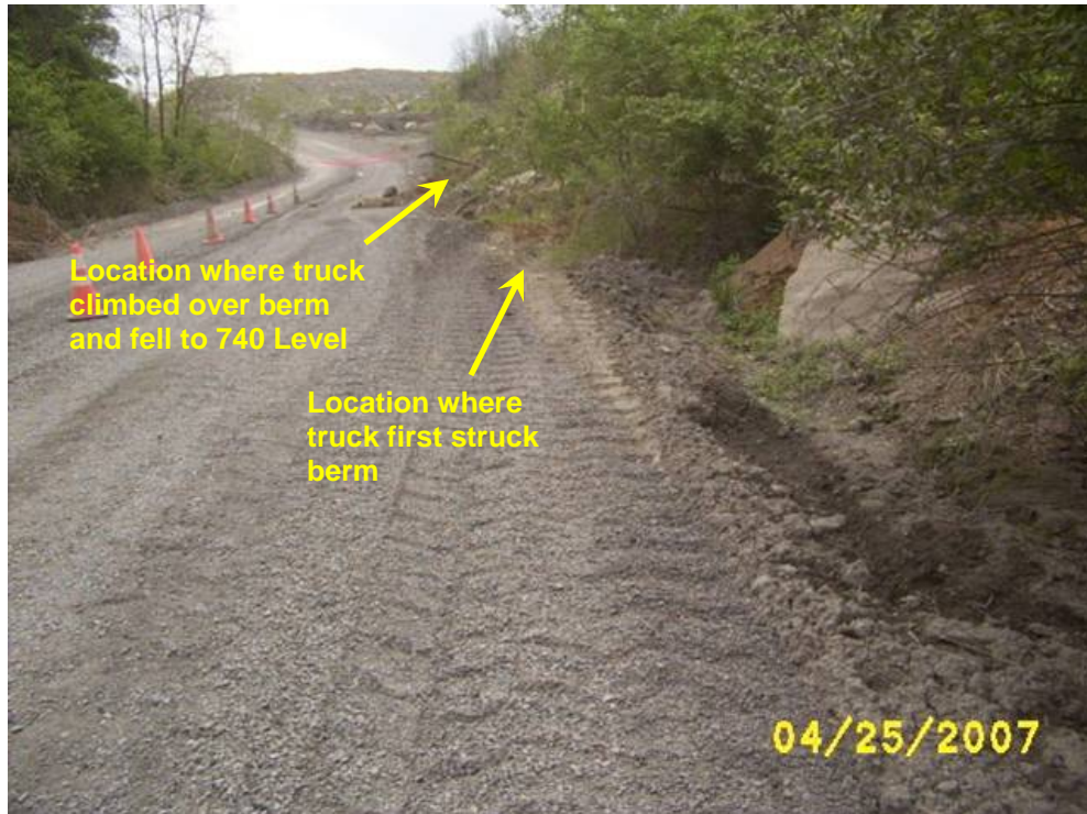
Figure 2 - Photo showing locations where truck left the haul road.
