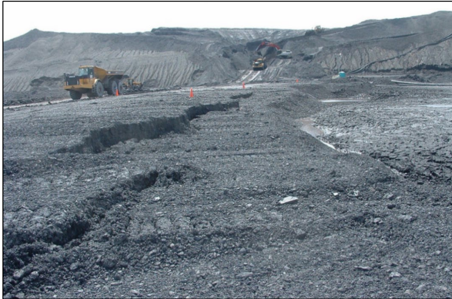
Photo 11. Failure of upstream pushout.
