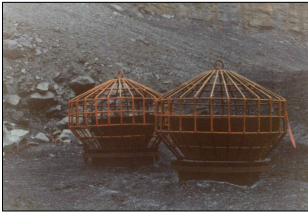
Photo 16. Trashracks on principal spillway inlets.
