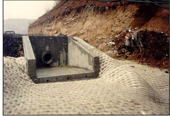
Photo 26. Headwall and concrete erosion protection at pipe outlet.
