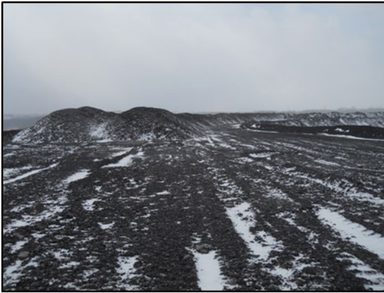
Photo 7. Poor placement and compaction.
