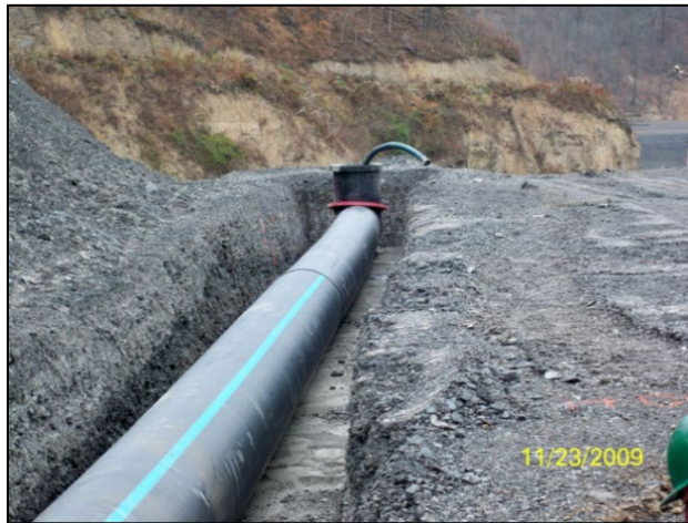
Photo 14. Principal spillway installation in trench.
