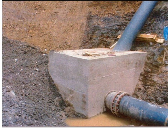
Photo 15. Thrust block at bend in pipe.
