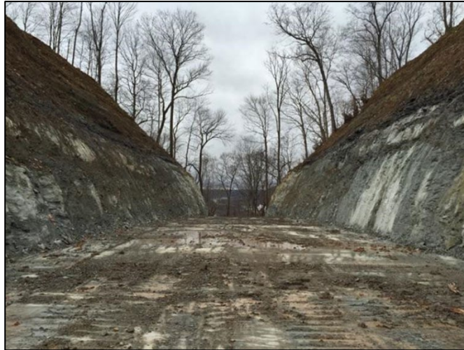
Photo 19. Open-channel spillway excavated in rock.
