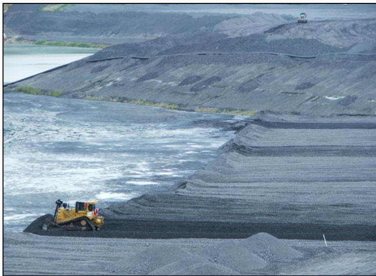
Photo 5. Construction of initial pushout at a coal impoundment.
