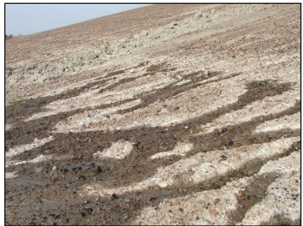
Photo 22. Seepage emerging on downstream slope.
