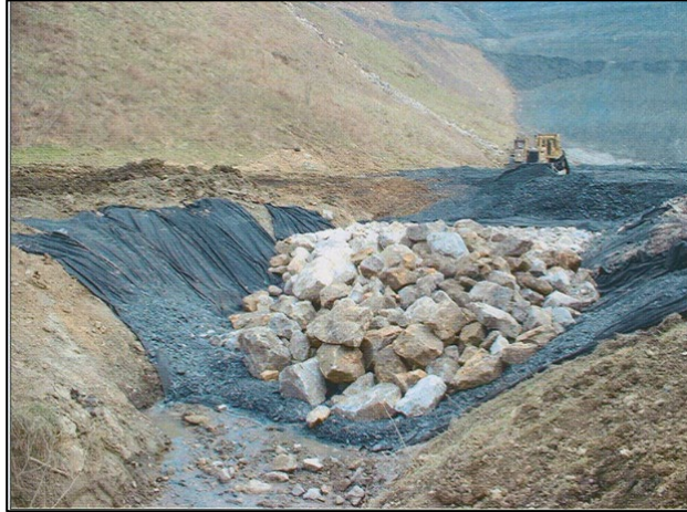
Photo 6. Construction of blanket drain. Note layer of cushioning material at bottom.
