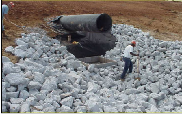
Photo 25. Construction of erosion protection at pipe outlet.
