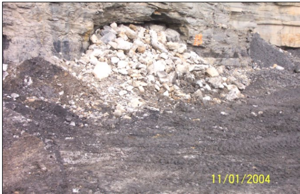
Photo 20. Backfilling mine entries.
