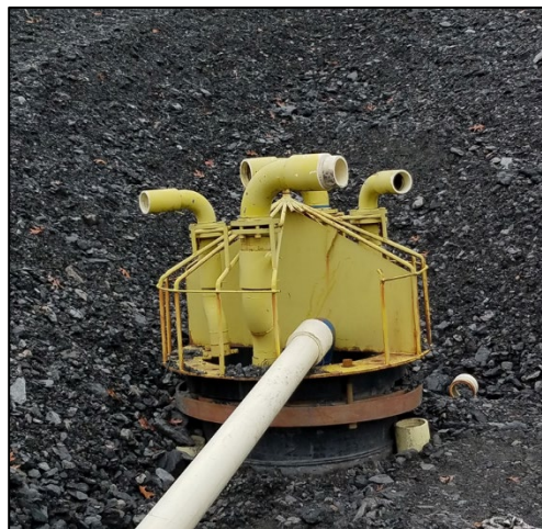
Photo 18. Pump lines inserted in principal spillway inlet.
