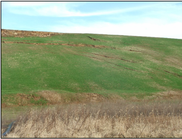
Photo 23. Cracks on embankment slope.
