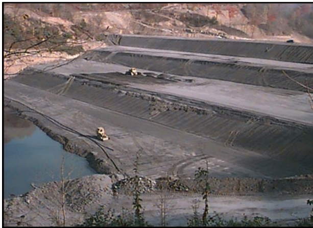
Photo 1. Construction of a coal impoundment embankment.
