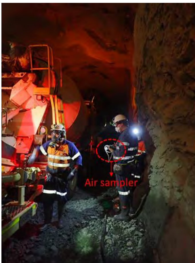
Figure 10: Air sampling during the Shotcreting activity.
