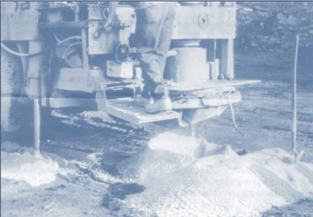
Figure 2. Drill operator at the control panel.
