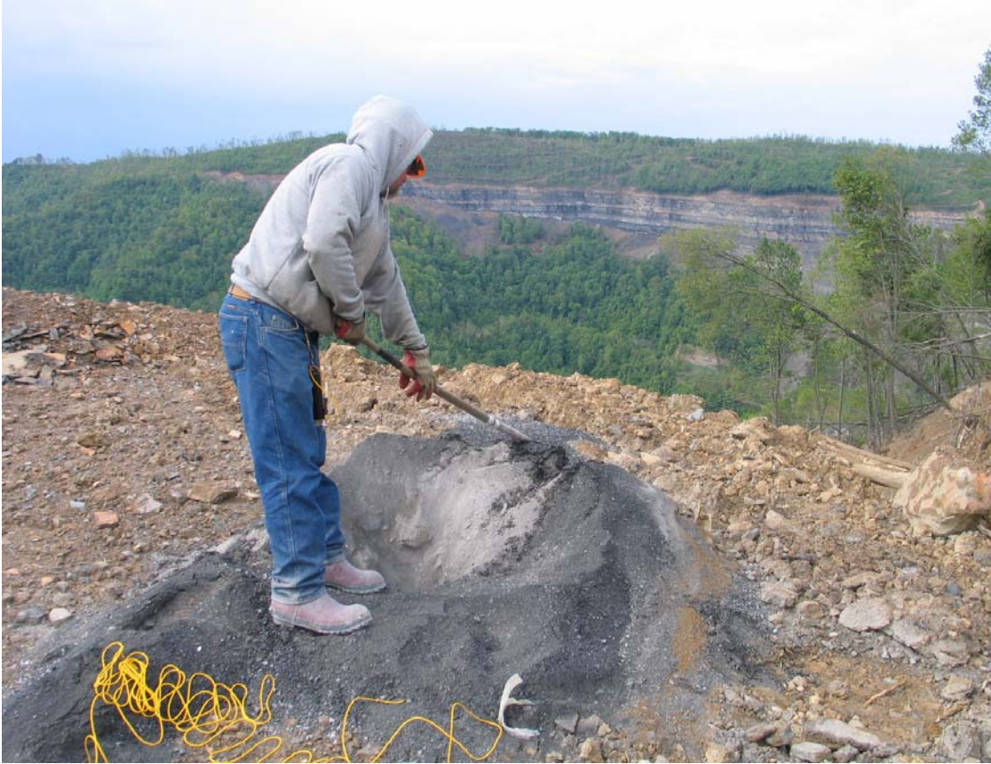
Figure 14 – Stemming a blasthole
