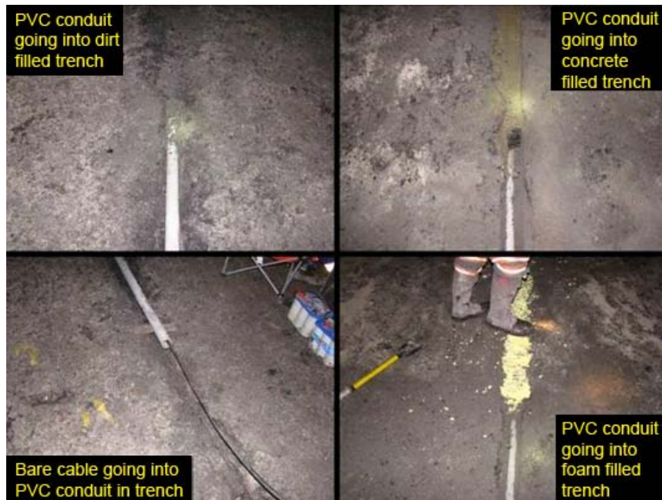
Figure 4-3. Examples of trenching conductors.
