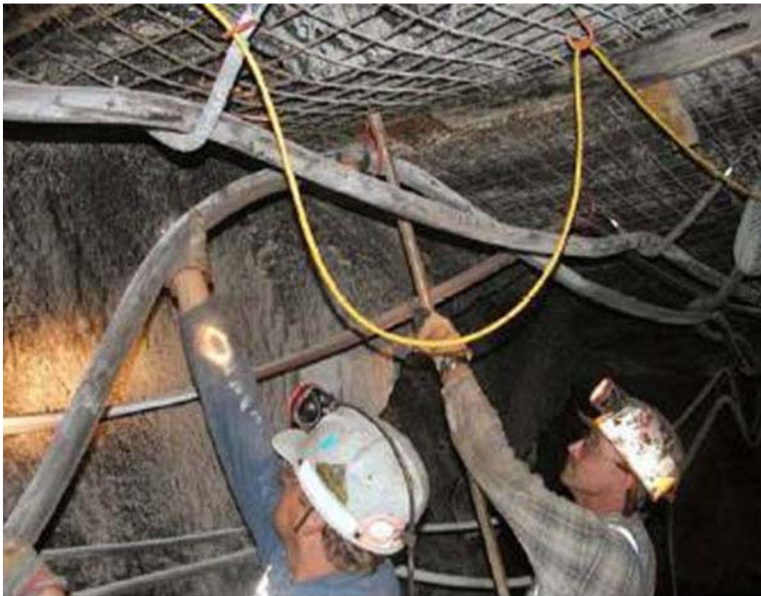
Figure 4-2. Hanging conductors from the roof.
