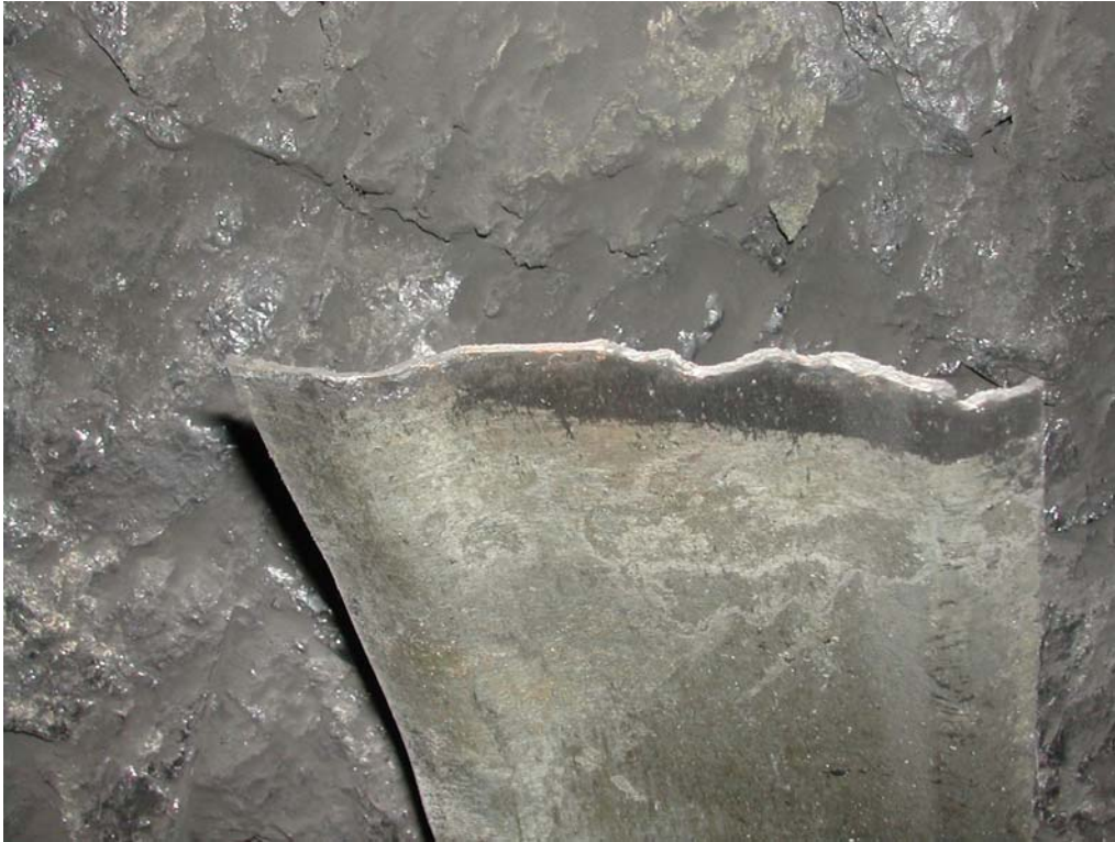
Photograph 5 - Inby segment of roof strap at A Left No. 3 Seal
