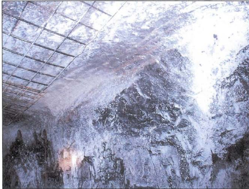
Photo 2. Minor Rib Sloughing at Crosscut 122 in the Second Entry from North Remnant Pillar
