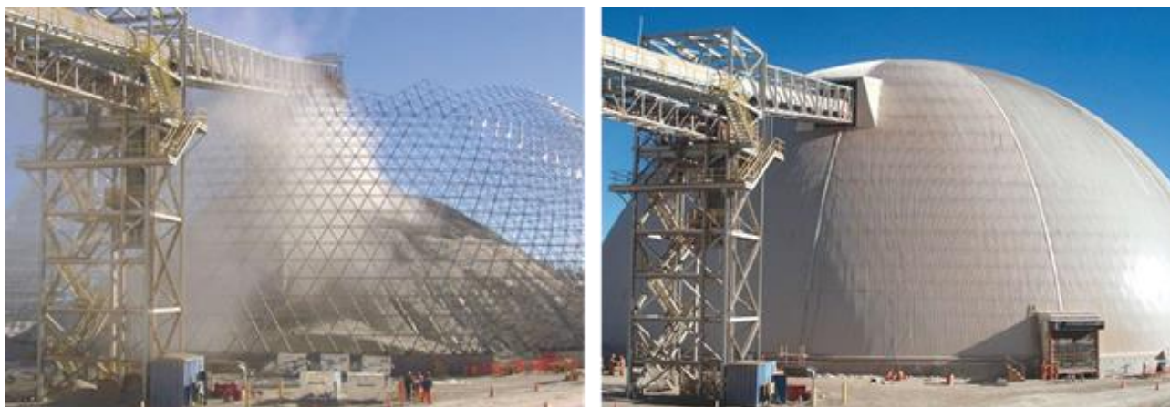
Figure 11.16. Photos of domes. The left photo shows dome construction while a stockpile is in operation and the resulting dust generation. The right photo shows the completed dome [from Walker 2016].
