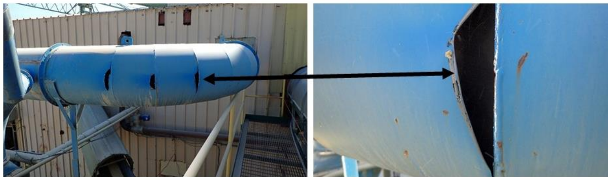
Figure 2.10. Photos showing multiple holes created along an elbow from wear and abrasion when a high-velocity system is used.
