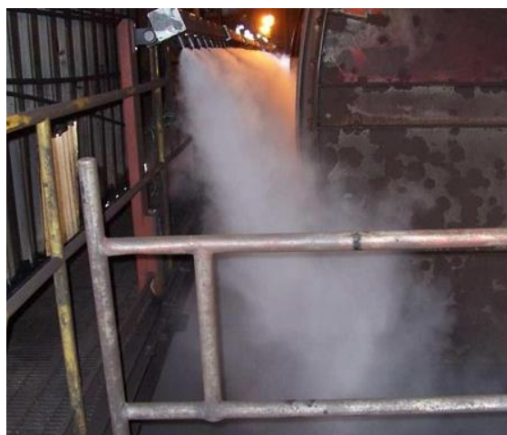
Figure 3.15. Typical dry fog nozzle spray patterns. The left photo shows sprays mounted above a grizzly at a railcar dumper. The right photo shows a primary crusher with nozzle manifolds.
