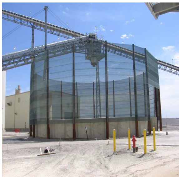
Figure 3.14. Typical wind fence installations. The left photo shows a porous windbreak material around a stockpile drop. The right photo shows the material being used at the top of a loadout hopper.
