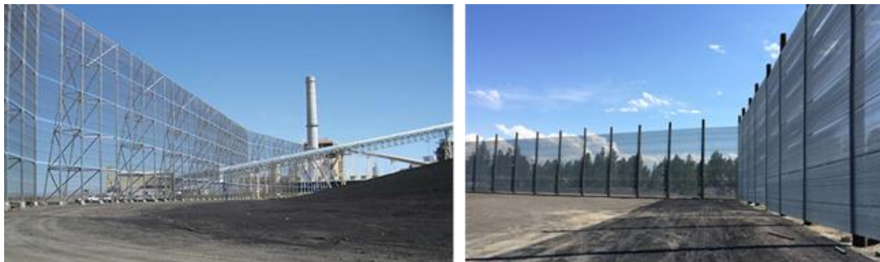
Figure 11.15. Photos of wind fences. The left photo shows a large wind fence installed at a coal power plant [from Larson 2015]. The right photo shows a more common size of wind fence.
