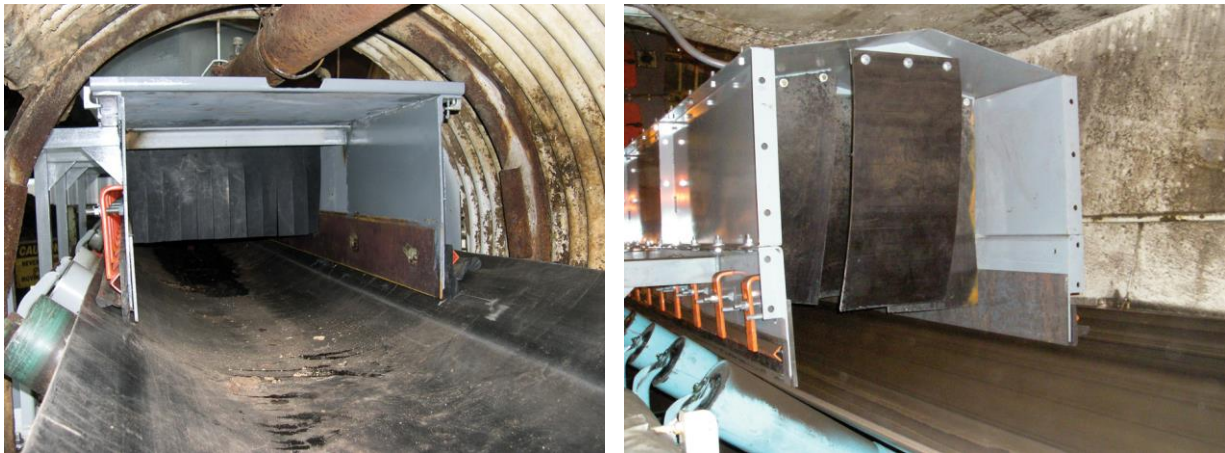
Figure 6.16. Exit curtain and intermediate curtain. The left photo shows an exit curtain designed to keep the dust and air inside the chute. The right photo shows intermediate curtains, which lengthen the route the air must travel and slow its velocity, allowing the dust to settle on the ore before being conveyed. In the right photo, the last section of the chute containing exit curtains has been removed for demonstration purposes.
