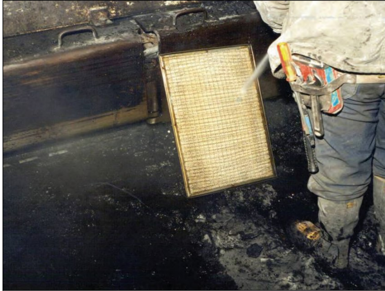
Figure 4-7.—Cleaning scrubber filter panel with water spray.
